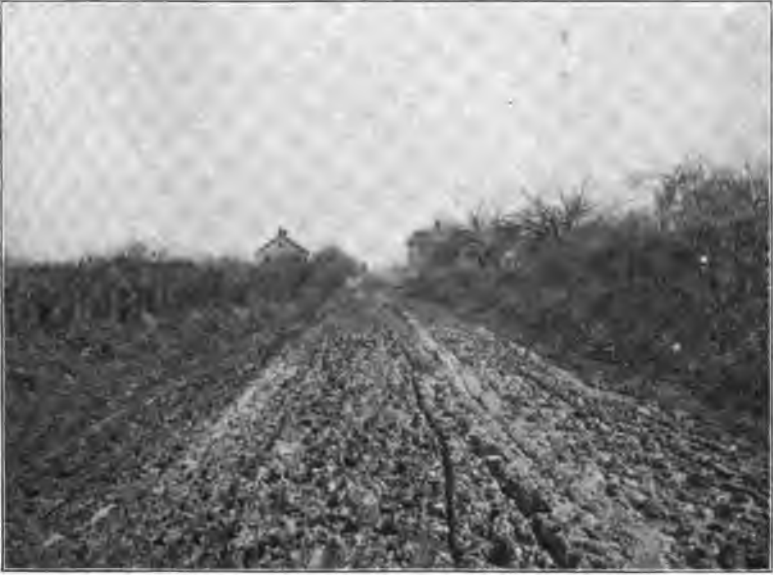
Neshanic road, Somerset Co., before improvement.
